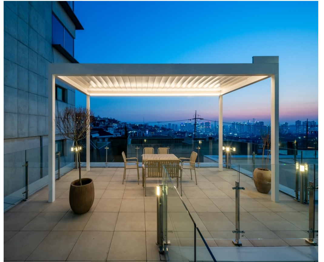
OSKA pergola installation — Seoul
